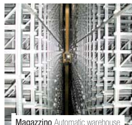
Magazzino Automatic warehouse
