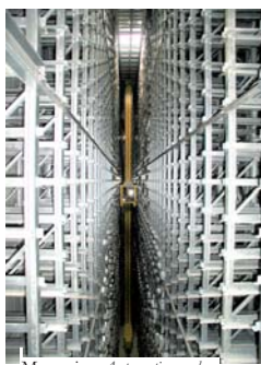
Magazzino Automatic warehouse
